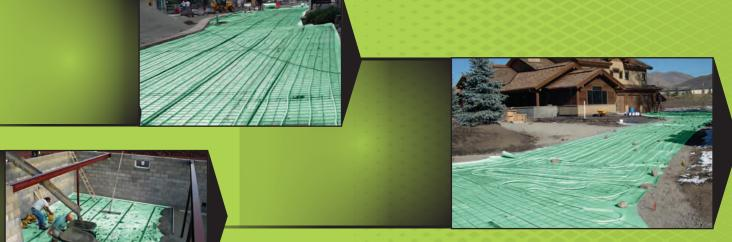
To provide greater comfort and energy efficient living, the easiest way to stop heat transfer between ground and slab, is to install LOW-E™ Slab Shield insulation.
