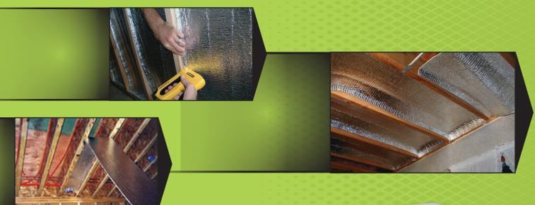
Low-E Tab Material makes installing ESP Low-E® Insulation in residential stud cavities as easy as can be. Low-E Tab is cut to 16" or 24" on center so it can benefit commercial buildings, structures with radiant heating as well as residential applications. The product is very easy to install and does not require special clothing or respirators to do so. The product is hypoallergenic and does not promote growth of mold or mildew.
