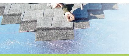
Therma Sheet Insulation may be installed directly under shingles. First install a standard approved underlayment as per the manufacturers directions. Next install Therma Sheet insulation as shown in the pictures below using the overlap flange as a rain drip edge. Shingles are then installed as per the manufacturers instructions.
